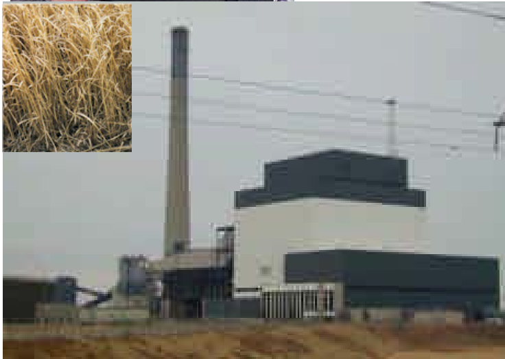
Ottumwa Generating Station – 750 MWe coal fired power plant that co- fires 17.5 MWe switchgrass
