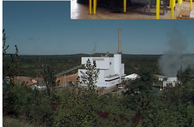
McNeil Generating Station – 50 MWe wood fired power plant
